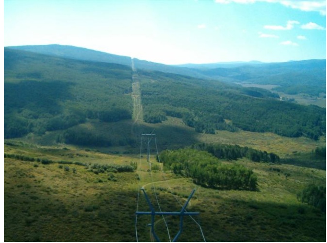
Transmission line in western Colorado
